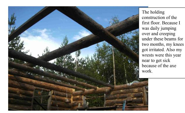
This log is crossing the wall and holding the balcony and the first floor. The gap on the upper side of the beam gives space to the logs to settle.
