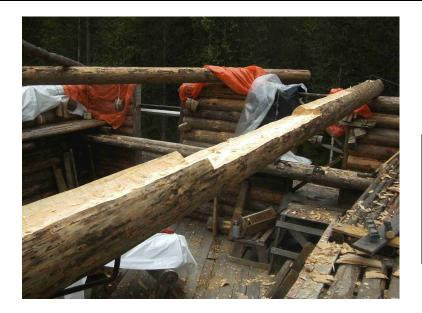
This is the profile of the log, which closes the gap above the windows and doors.
