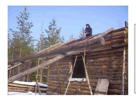
This way heavy logs can be lifted easily. The rope is fixed to the wall. The rope turns around the log and returns back to my hands. This arrangement makes the effort of pulling two times lighter. The ramp is also making it lighter.
