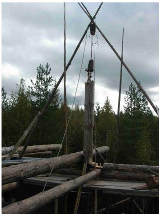
With the pully a placed the posts, which are holding the long roof beams: each 12 meters and about 350 kg. I had to turn them into the right direction.
